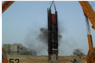
Closed End Diesel Hammer
