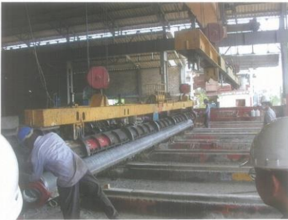
after curing, Cutting the PC wires and Demolding
