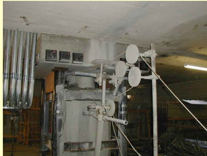
Cutting column prior to isolator installation
