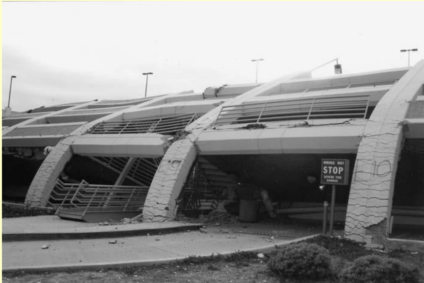
Parking structure that collapsed during the 1994 Northridge earthquake, California
