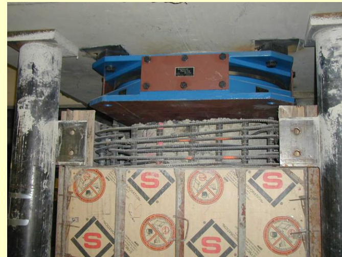
View of isolator before column below cast
