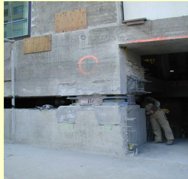
Isolator installed in exterior wall
