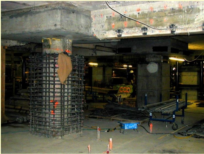
Rebar cage around basement column
