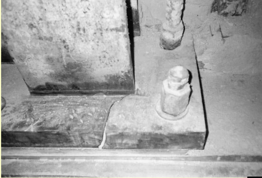
Cracks in 4-in.-thick base plates during the Northridge earthquake, Oviatt Library Annex Building
