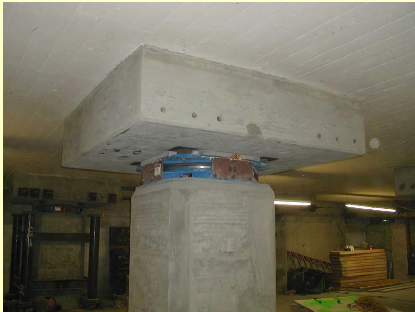
Completed isolator installation atop interior column
