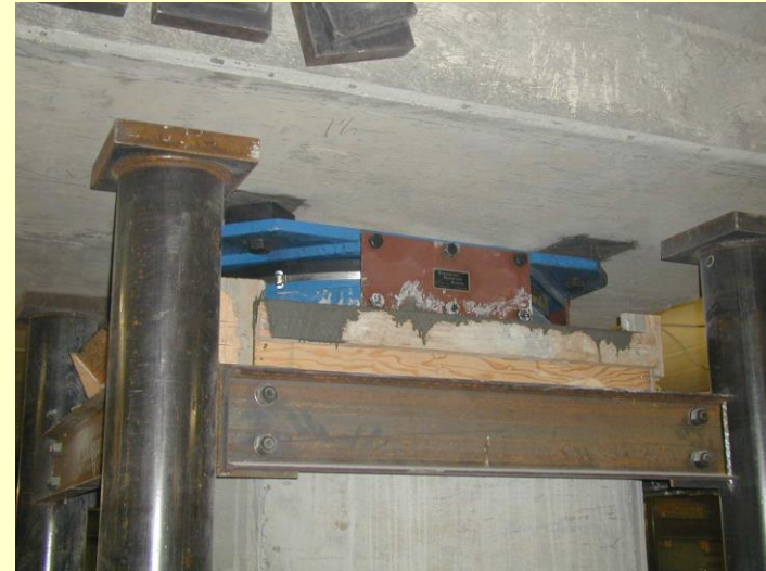
Grouting to underside of isolator
