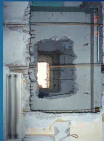
Debris shaft formed by opening temporarily cut on floor slab
