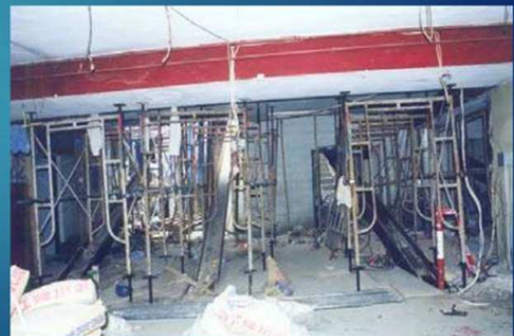
Temporary props erected to support heavy equipment
