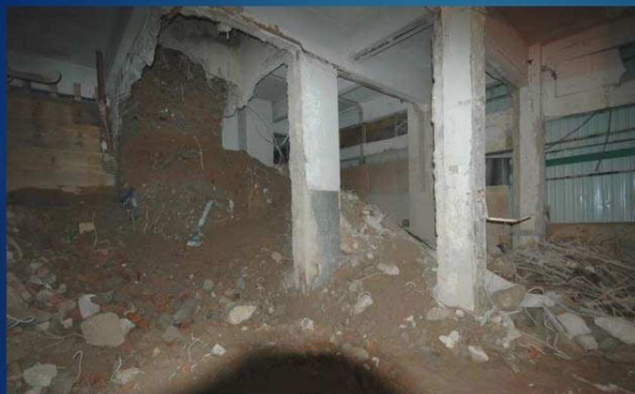
Debris collection area at ground floor under the debris shaft
